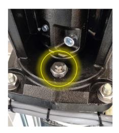
The coupling guard will need to be removed to gain access to the bleed screw.
